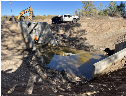
Another view of the internal kettle area.
